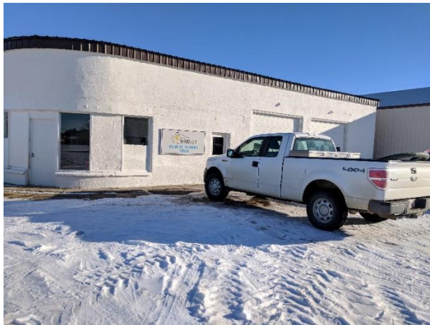
Figure 11 - Warner Public Works Shop
